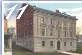
11 Ossining Municipal Building 1915
